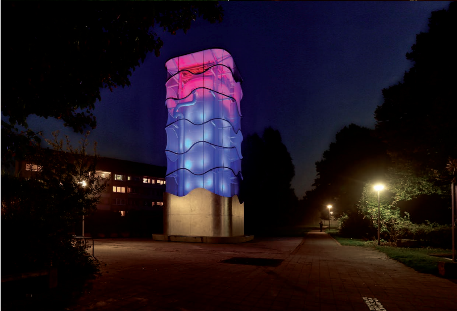
Wärmespeicher (Germany) Photo Credit: SSP Design
